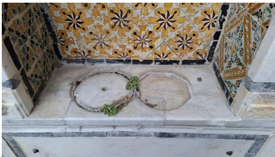
Fig. 9. Photograph of the cistern opening in Dar Othman, Medina of Tunis, 2025.
